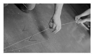
Measure an even distance from two points on the wall and mark the floor. Run a chalk line between the marks and flick the line.
